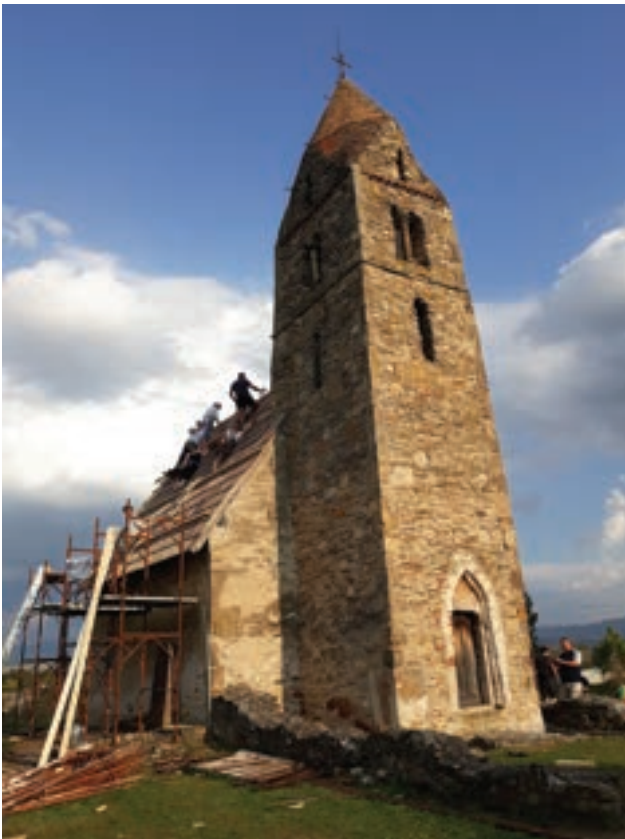
▲ Fig. 5. The medieval church in Strei during the roof intervention.
