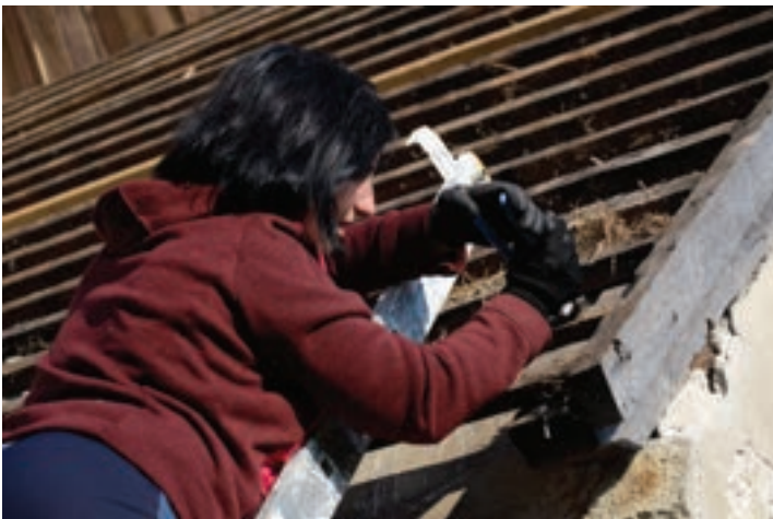
➤ Fig. 22-26. Snapshots taken during the 'Ambulance for Monuments' intervention: dismantlement of the old roof and renewal of the exterior open drainage ditch.
