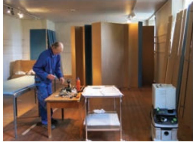
Fig. 9: A small section of the wall system mounted on the 18 th of September 2015.
